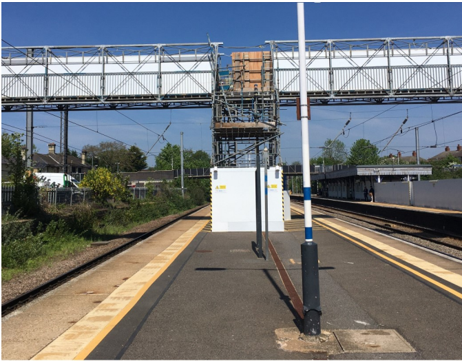
Close up of the temporary shaft to bring work staff and materials to a safe working space. Passenger trains pass the site on the centre tracks very frequently and at very high speed. Very long and heavy freight trains pass by on the outside tracks frequently at full line speed... the dust flies!
