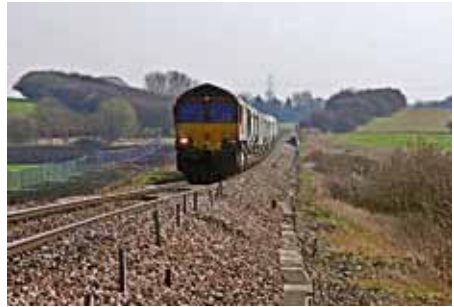
A candidate for the second track; marshy, fragile land between Stuntney and Ely approaching the River Ouse bridge. CB
