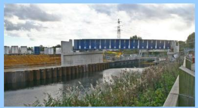
The photograph shows the first stage of the new bridge over the River Gipping at the eastern junction of the Ipswich Chord. The completed bridge and connection is due be installed during Christmas track possession. The final connection, to the main line north to Haughley is due for
