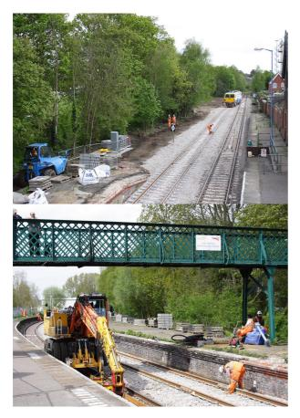
AT LAST, after many, many years of lobbying by both our Branch and the East Suffolk Travellers Association (ESTA), Network Rail has descended on Beccles station and installed the much needed loop and associated signalling. Most of the work had been completed by 13 May ultimately making possible the hourly rail service expected in the next timetable change in December.
