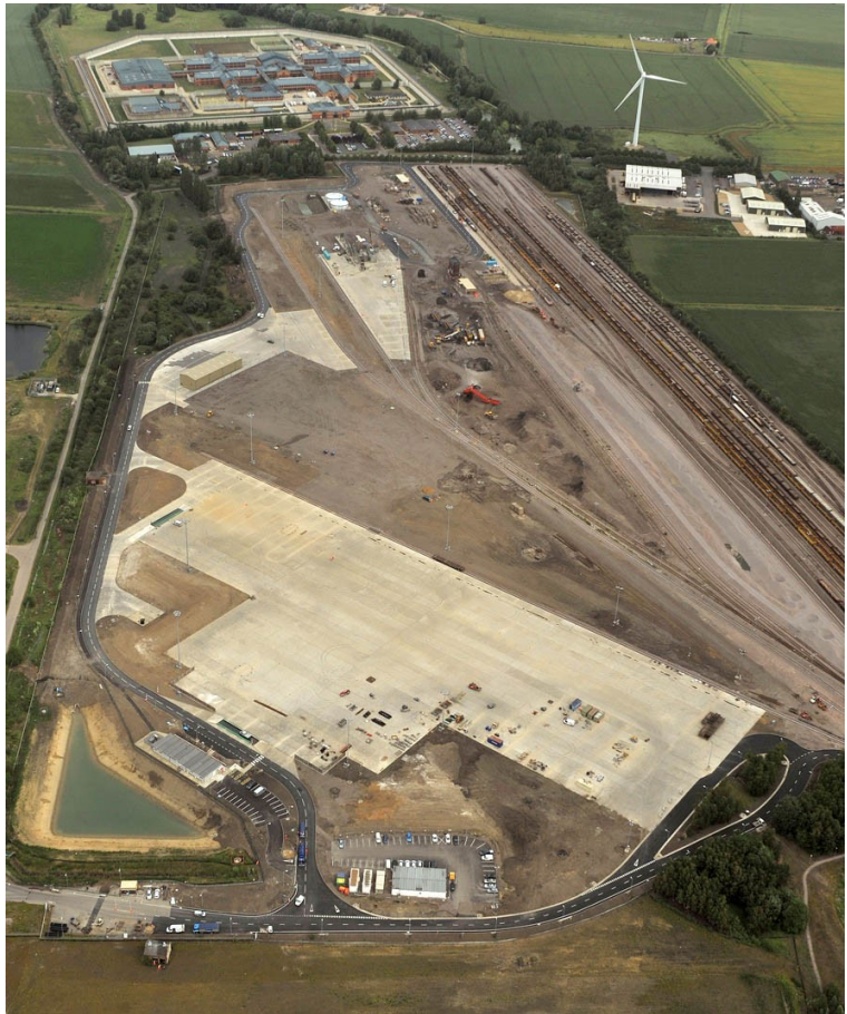
March, Whitemoor Yard showing new recycling centre. Photograph courtesy Network Rail
