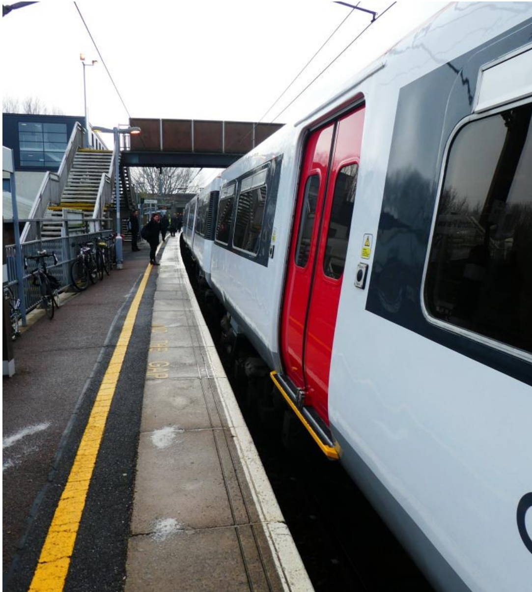
Picture 6(A): The up platform. There is a large gap, both in height and distance between the platform edge and the train.
