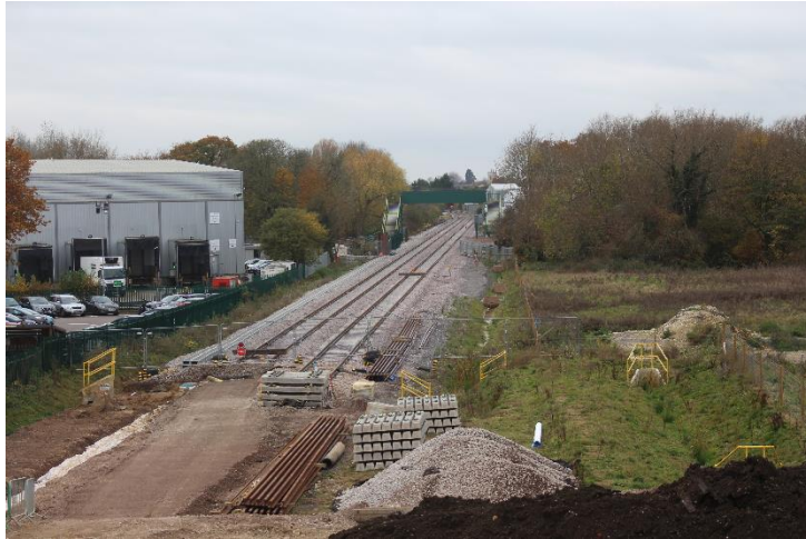
Towards Bicester from Charlbridge Lane Bridge (new)
