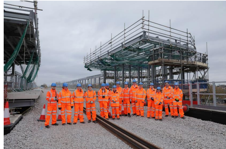
Bletchley Flyover with High Level Station
