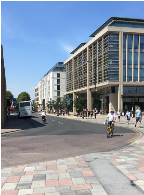
Picture 2: The pedestrian area leading into Station Road and the historic City Centre. This broad pavement leading from the station entrance provides a traffic free walk for a considerable distance into town.
