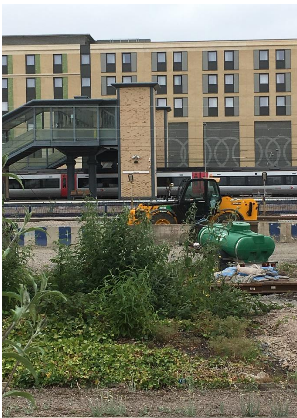
Picture 4: Looking from Clifton Road to the existing north end footbridge. This will be extended eastward to new platform 9/10 when it is built.
