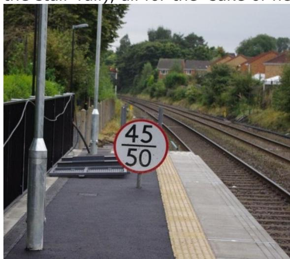
this on Hednesford platform 1? It needed to be extended to take 4-car Class 170s trains. At the end of the old platform there was a speed restriction sign. Rather than move the sign to the end of the new platform the new platform has been built around it. Not only was it a trip hazard, but drivers would fail to be reminded of the speed restriction owing to passengers obscuring the sign.
