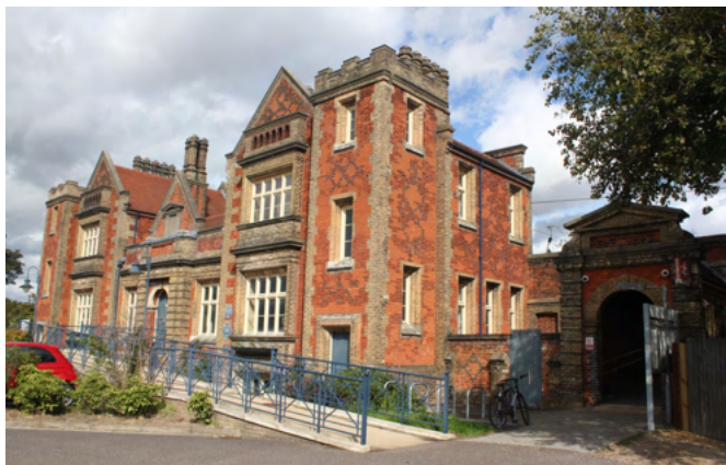
2018: The station at Needham Market, Suffolk, was built in 1846 to the designs of Frederick Barnes. His grand battlemented offices are no longer used by the railway so entrance to the platform is through the arch on the right Picture by Geof Sheppard
