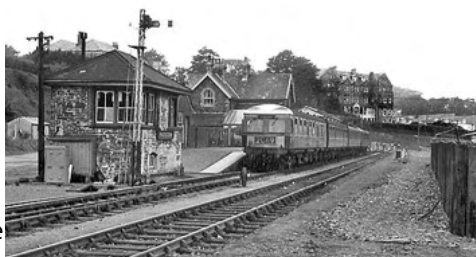
Padstow station in 1965. Closed in 1967 against TUCC advice
