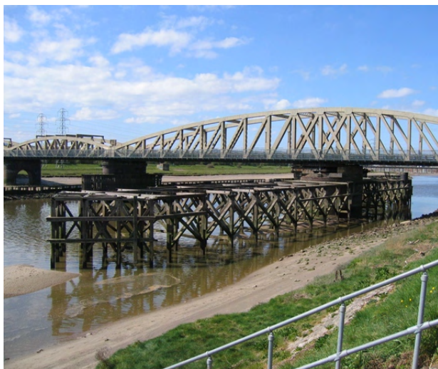
Hawarden Bridge over the River Dee still (in 2022) carries the Wrexham to New Brighton railway over the river, and at one time used to swing open for tall shipping. There was strong resistance when BR wanted to close the line in 1965
