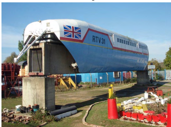
PRESERVED: All that remains of the Tracked Hovercraft test system, the RTV 31 test vehicle and a single portion of its guideway preserved at Railworld, Peterborough
