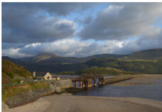
Barmouth Bridge, probably the most significant piece of infrastructure on the Machynlleth-Pwllheli route, has been closed temporarily several times since 1967 to allow repairs which were still ongoing in 2022
