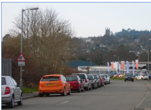
Photo 4. The North Cornwall Line a ¼ mile short of the former station with the main single track running line marked by the pavement on the right (north) side. The radius here was 18 chains (360 m). The left hand pavement and adjacent land (on a former siding and head shunt) would be best used for a new running line as fewer entrances would be blocked. The church on the hill is St. Stephen's. View WNW.
