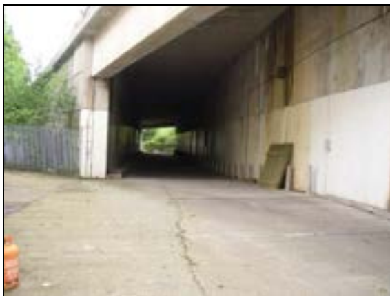
Figure 9: Tunnel Under M40
