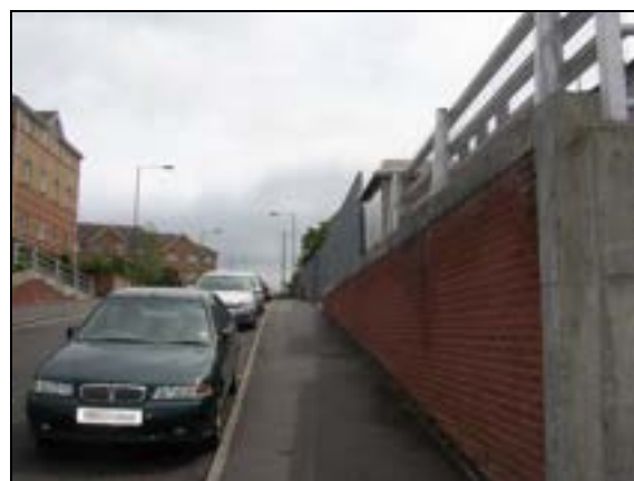
Figure 4: Princes Gate looking south-east
