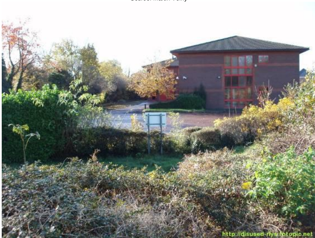
Figure 41 - shows the proposed HULTS alignment in Bourne End area and detail of the Boston Drive business centre built on the original rail alignment.
