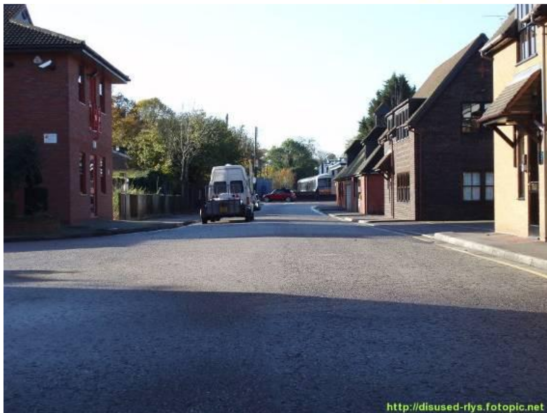
Figure 42 - shows the proposed HULTS alignment in Bourne End area and detail of the Boston Drive business centre built on the original rail alignment.
