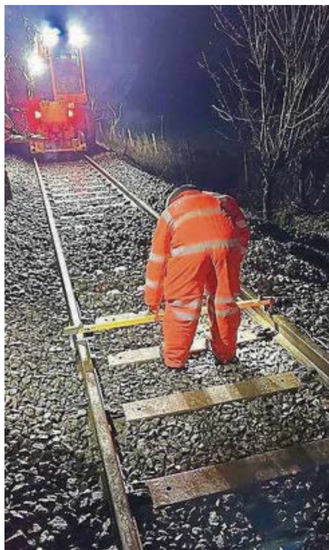
Maintenance and repair work on the Tarka Line
