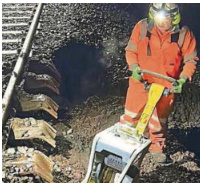
Night shift working to fix washouts between Crediton and Cowley
