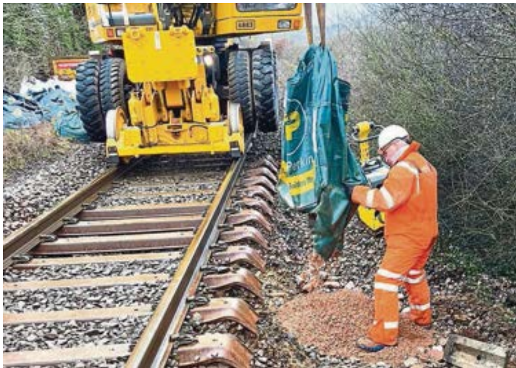
Engineers pictured working to fix washouts on the Tarka Line between Crediton and Cowley
