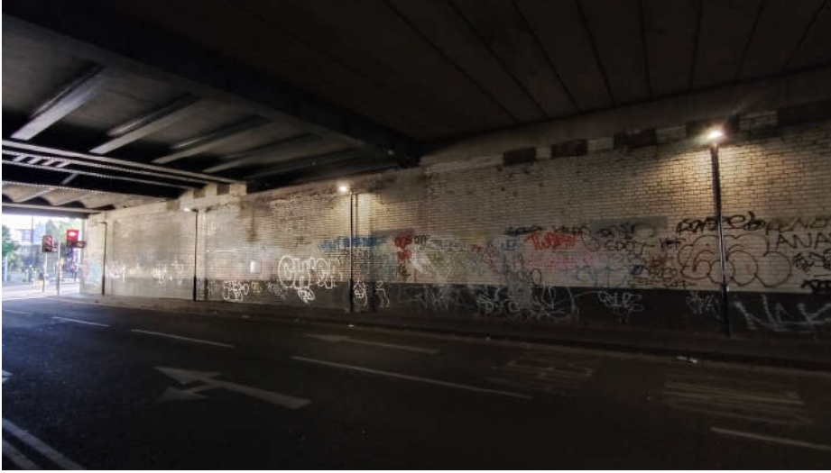
Park Street (undercroft)
