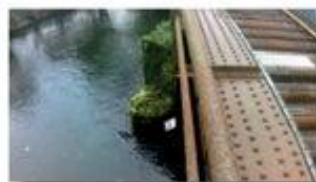
Above, the white marker is the flood alert level and below, the same bridge parapet underwater - photos courtesy Network Rail
