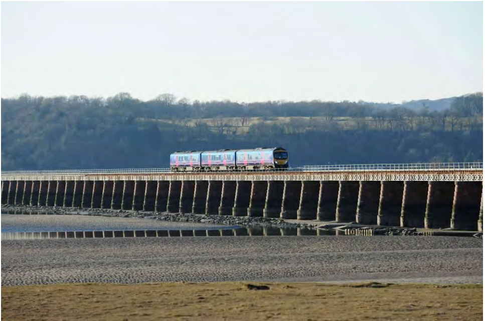
Arnside Viaduct with a Trans – Pennine Express class 185 crossing. Photo courtesy Network Rail
