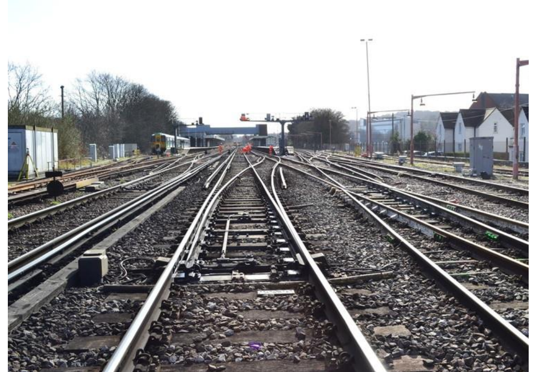
Engineering work during Redhill platform 0 construction , Arup
