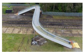
Go with the F.L.O.W. (Fibre reinforced polymer, Low-cost/Light-weight, Optimised design, 'Working' bridge)
