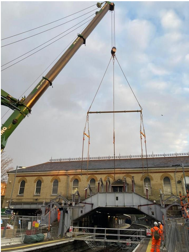
Out with the old at Chatham – completion due Spring ’22
