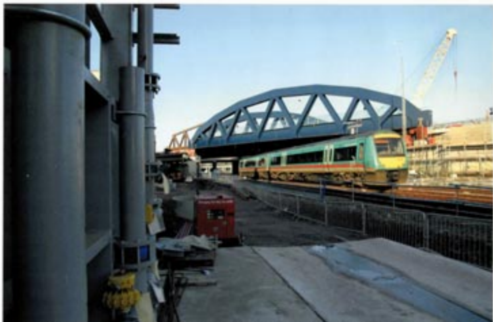
(Picture Rail link Engineering) A new bridge for the Channel Tunnel rail link over the midland main line outside St Pancras with Class 170 below. These units have pioneered improved services and will soon be replaced by higher capacity trains. Below is a European high speed unit which has helped to take significant traffic away from the airlines
