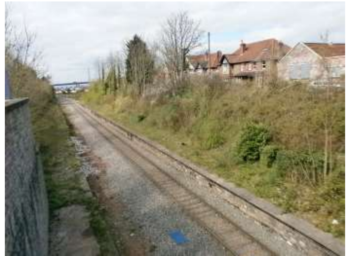
The existing Portbury freight line at Pill station will remain and a second track will be laid on the left for passenger trains to/from Portishead. Photo by Nigel Bray
