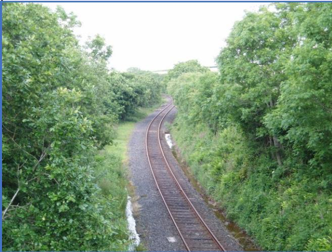
*Photo 4. Looking north from farm overbridge 605. The platform would be on the left side. On the right the flooded section up to the middle of the picture is thought to be level track. Beyond, it is 1 in 88 down towards Crediton. (2012 photo)*
