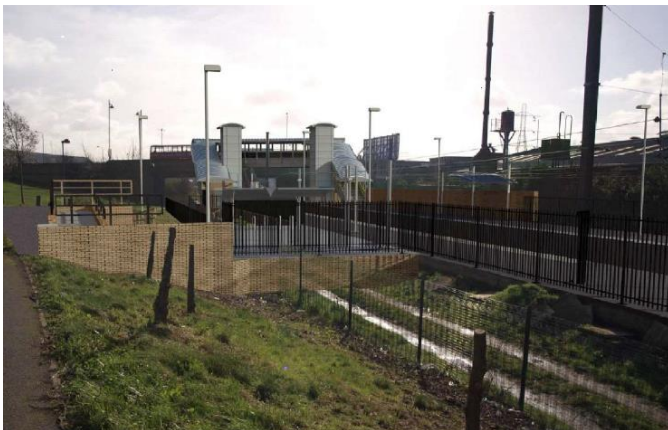
Lea Bridge station – looking south, towards Stratford
