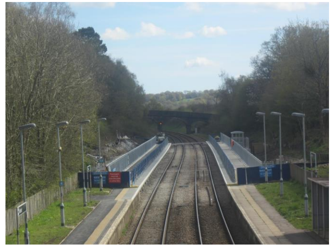
Platforms at Ashurst extended by 114m, looking south
