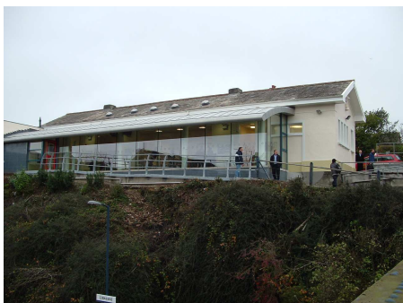
Refurbished Liskeard station with its new station buffet overlooking the platforms.
