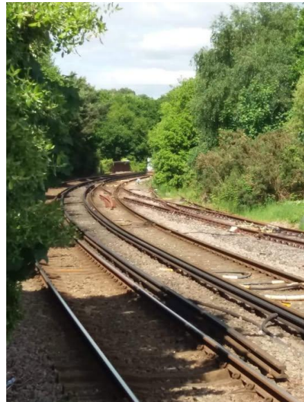
Renewing the crossover onto the Hamworthy branch in May 2022
