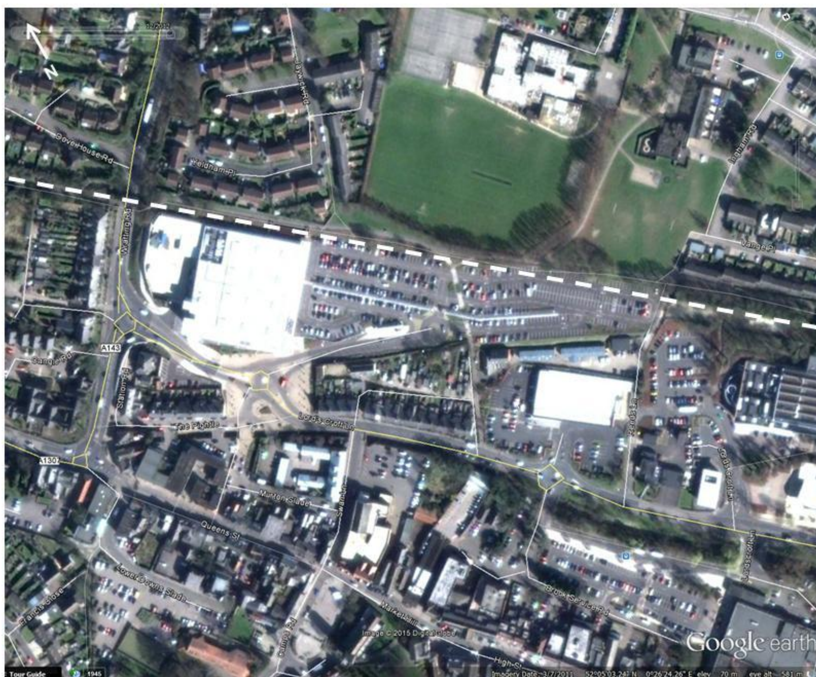
Figure 14: Haverhill (Town Centre)
