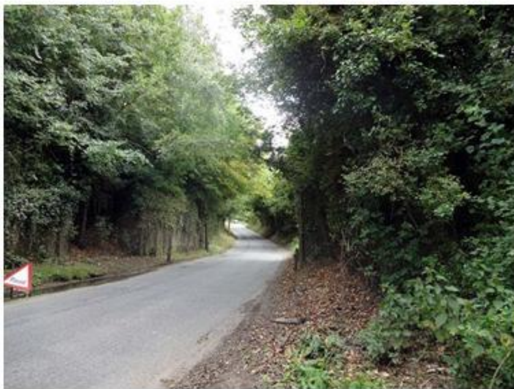
View south-west, showing abutments
