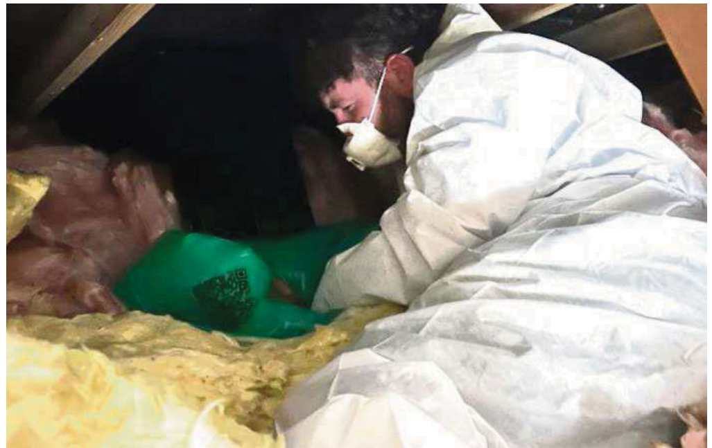
The ARC Eaves Insulator being fitted
