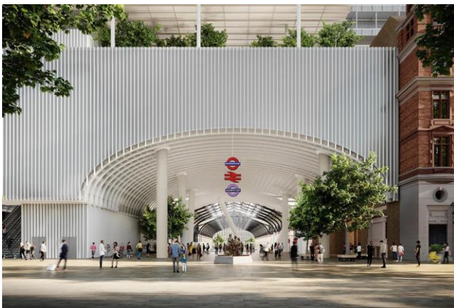
Liverpool Street side, looking north
