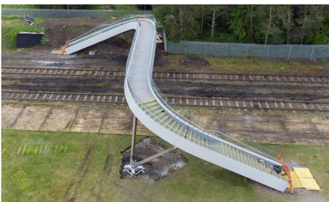
Go with the F.L.O.W. (Fibre reinforced polymer, Low-cost/Light-weight, Optimised design, 'Working' bridge)
