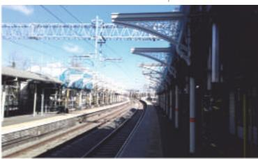
Connection point: Kettering station, looking north on the fast lines. Electrification covers all four lines through Kettering, though the electric 'Connect' services will use the slow line platforms, behind the buildings on the right. A consequence of electrification is that the ornate iron canopies are being modified and handsomely restored. This view shows work in progress on 6 April 2021.
