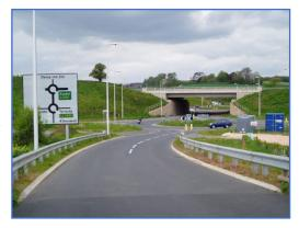
The chord on straight track could pass under the bypass road bridge in the background and on the left (south) side. It would be necessary to cut and divert the two roads leading left off the two roundabouts also visible on the road sign. Continuing at 240 m radius the Plymouth line could be rejoined in about a ½ mile (360 m) and to the south of the Old Kingskerswell Road bridge (railway location 215 m 46 c).
