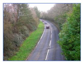
View SE from Ashburton Road, Bovey Tracey along the A382/ former railway. The green strip is wide enough to restore track to a new Brimley Halt on the left.
