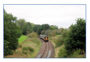
1) The 12:20 Waterloo to Exeter St. Davids on 15<sup>th</sup> October 2018 recedes into the distance as it rounds the sharp curve at Talaton. All the way from Honiton to Pinhoe it was the down line that was retained, but here the track is swinging on to the up formation to ease the curve (on the right).
