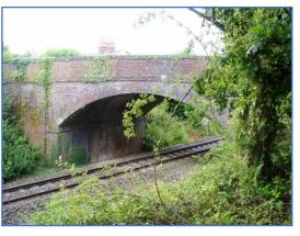
2) Bridge 499 between Talaton & Whimple shows how the arch design may restrict clearances for double track restoration.
