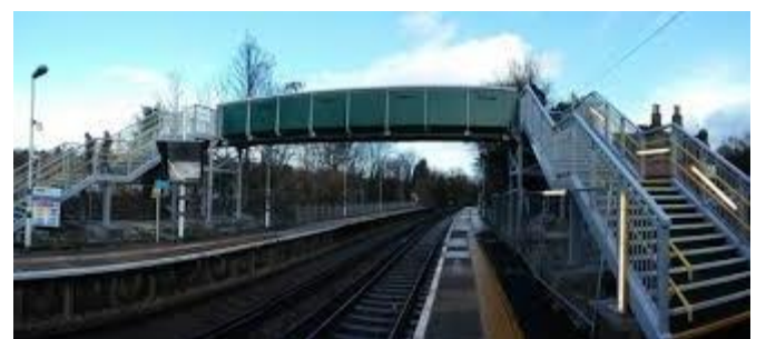
Reedham (Surrey): modern footbridge - passive provision for lifts?
